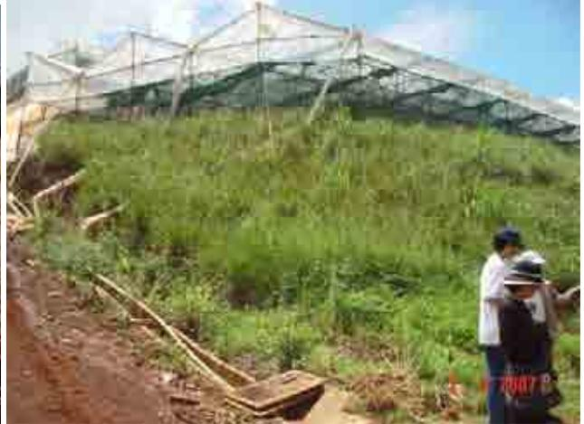
*Stabilisation of fill slopes created for glasshouses and at the same time absorption of nutrients in runoff from flower beds*
